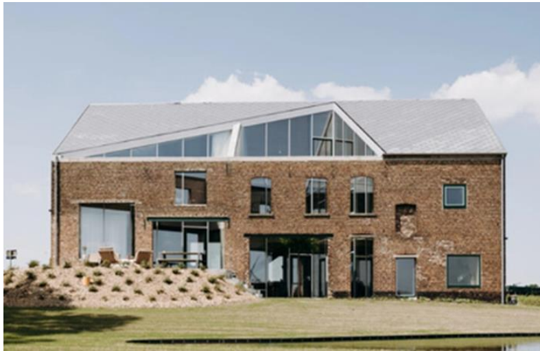
Figure 1: A building made of Rice Husk-based bricks.
